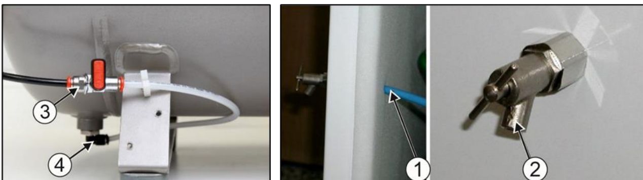
Fig. 7: Installation of condensate drain valve on cabinet
